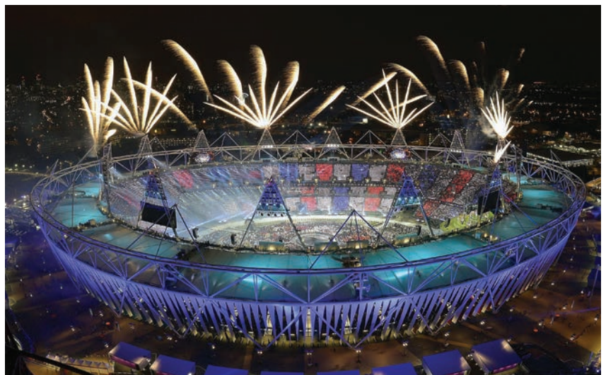
Cooley Group worked with Dow to develop the stadium wrap for London’s Olympic Stadium, containing the 100% recyclable Enviroflex polyethylene-based print media. It is printed in UV-curable inks, which contain little or no VOCs (volatile organic compounds)
